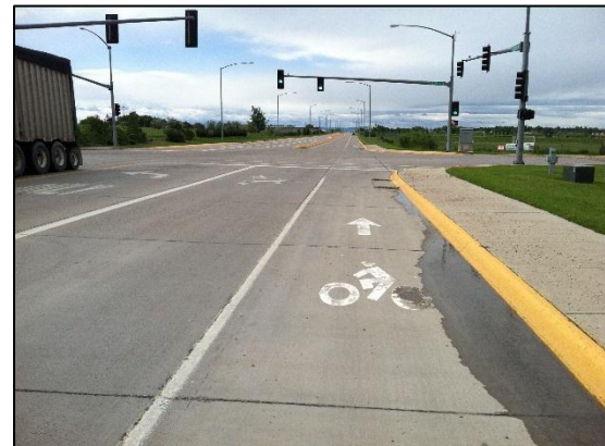
57 th St N/2 nd Ave N bike lanes, installed Summer 2013
