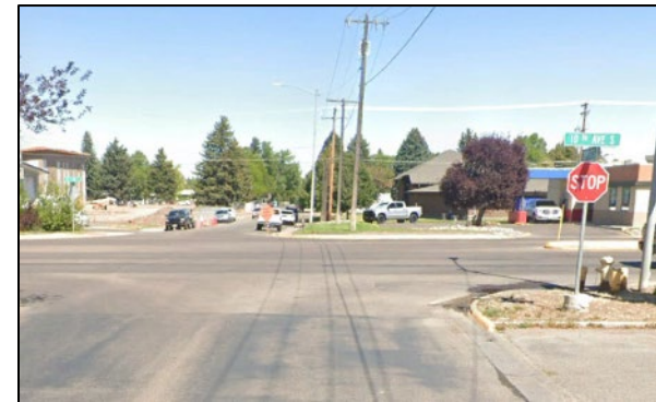
The intersection of 10 th Avenue South and 29 th Street South is two-way stop-controlled.
