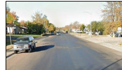
36 th Ave NE serves as a collector street for the North Great Falls neighborhoods.
