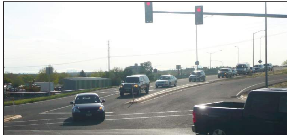
Poor intersection function at the intersection of I-315 Eastbound Off Ramp and 14th St SW can cause vehicle delays on the connecting roadways.
