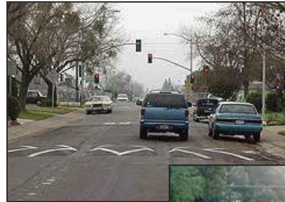
Raised Speed Bumps
